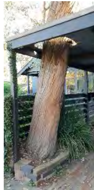
Trees in urban areas should be saved wherever possible; a carport has been added over existing hard landscaping and the tree has been incorporated in the design
